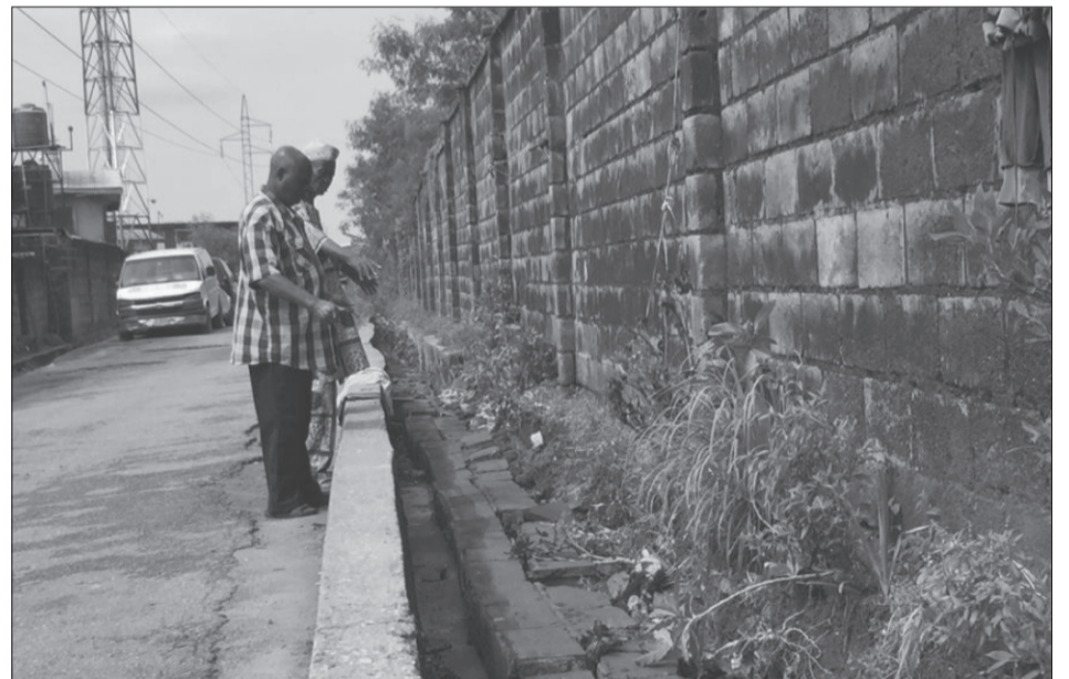
Fabukade CDA gutter collapsed after heavy rain at night
